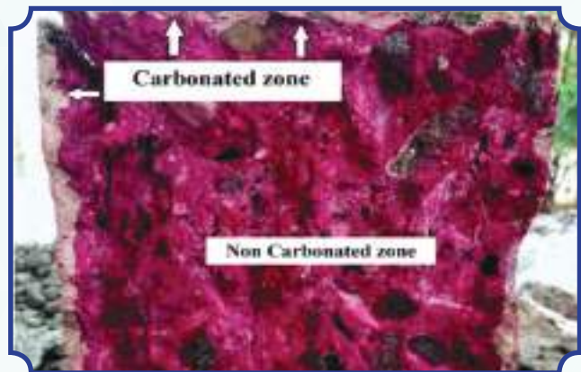
Carbonated and non- carbonated concrete
