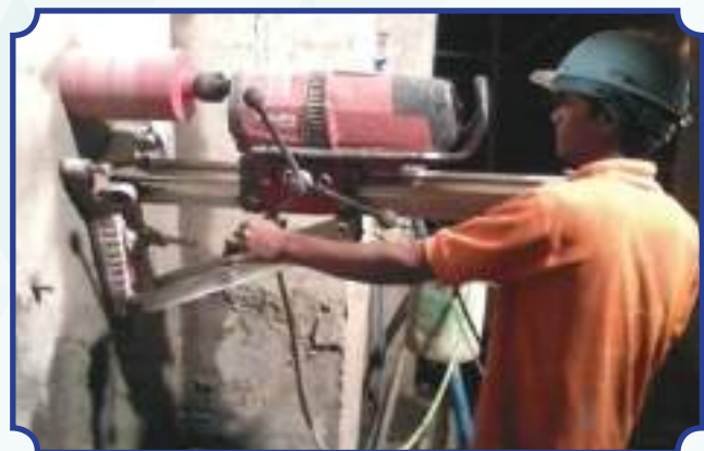
Core extraction in concrete.
